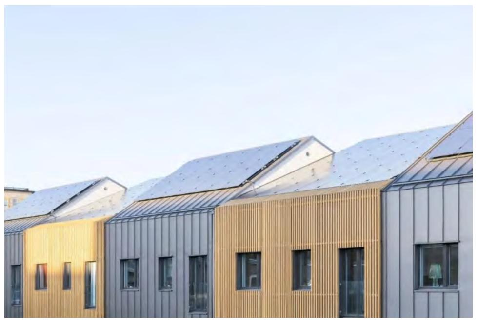
Power of 10 (Net zero energy home; passive house standard), Orebro, Sweden (cold), 148m2 / home, 0.4MWh/yr/home, 40kW battery. Street Monkey Architect
