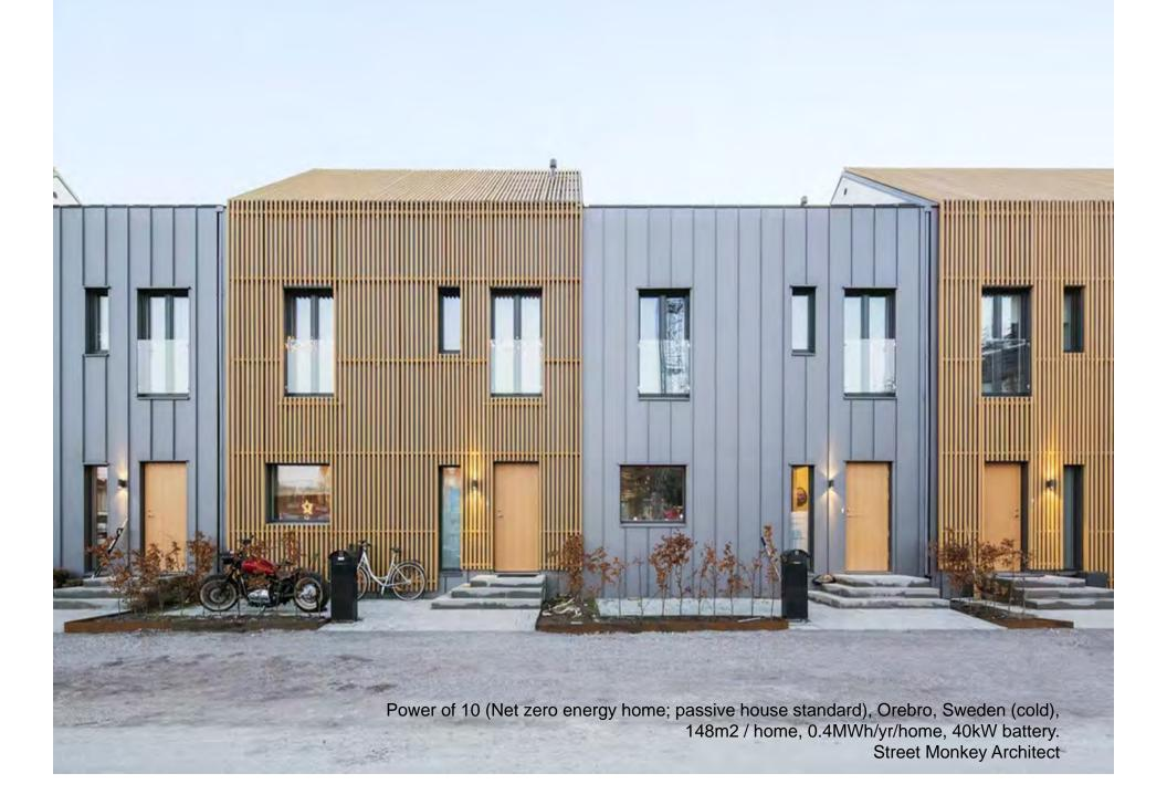
Power of 10 (Net zero energy home; passive house standard), Orebro, Sweden (cold), 148m2 / home, 0.4MWh/yr/home, 40kW battery. Street Monkey Architect
