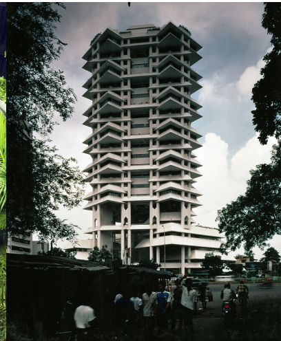
Wisma Dharmala Tower Jakarta, Indonesia | Paul Rudolph
