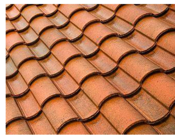
Recycled rubber roofing
